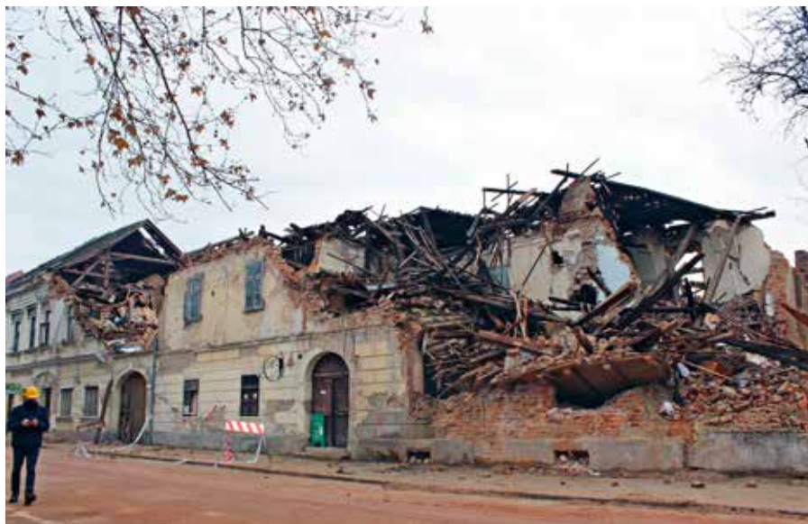
8 Posljedice potresa u Petrinji 29. prosinca 2020. (foto: T. Petrinec) Consequences of earthquake in Petrinja on 29 December 2020 (photo: T. Petrinec)
