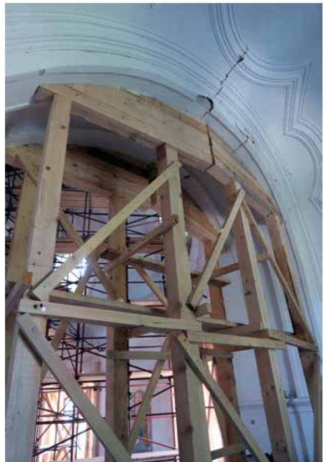
23 Shoring of the arch above the upper-choir which supports the nave vault (photo: X. Romão, July 2021)
