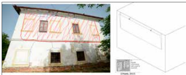
19 Out-of-plane mechanism n°2 in the east façade (photo and drawing: Thibaud Maillard, 2023)
