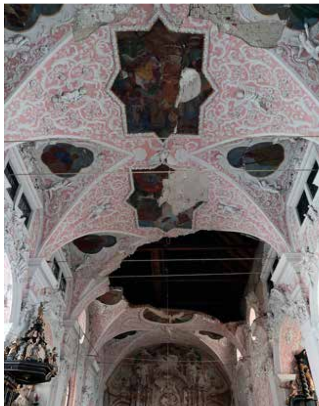
10 Longitudinal cracking along the vault crown line (photo: X. Romão, July 2021)
