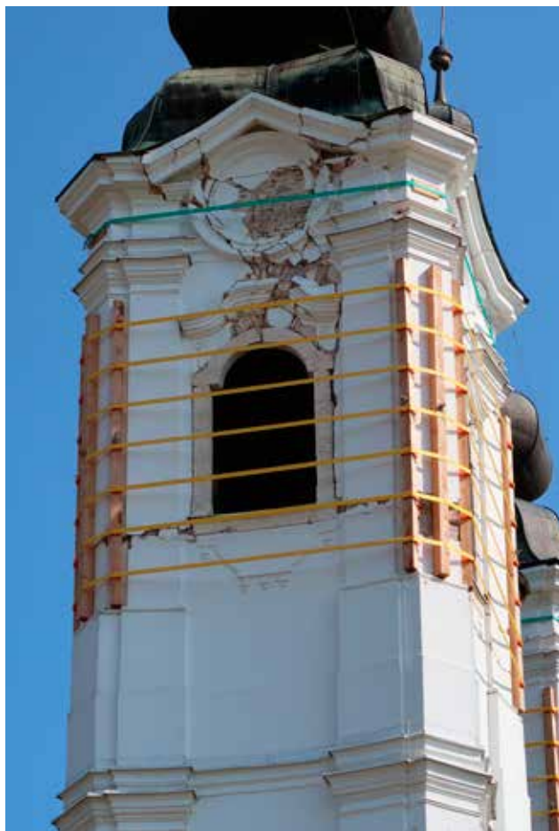
24 Damage in the upper zone of the tower (photo: X. Romão, July 2021)
