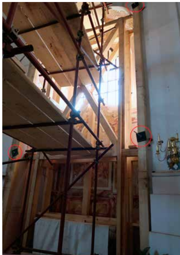
18 Detail of the internal shoring of the lateral chapels and anchorage connections to the exterior (photo: X. Romão, July 2021)
