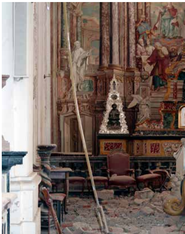
9 Detail of the failure of the triumphal arch tie rod (photo: X. Romão, July 2021)
