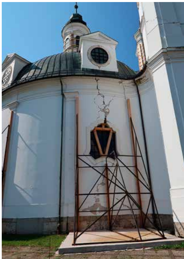
17 External shoring of nave walls in the area of the lateral chapels (photo: X. Romão, July 2021)
