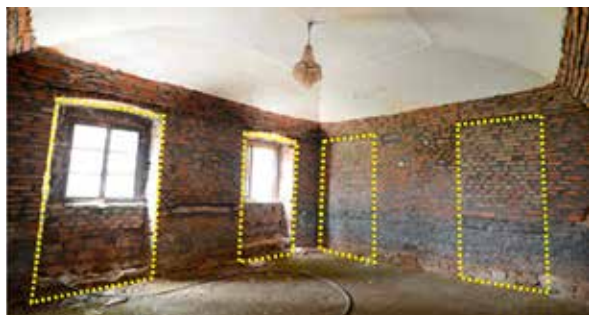
8 Examples of infilled masonry portions considered as openings in the EFM (photo and drawing: Thibaud Maillard, 2023)
