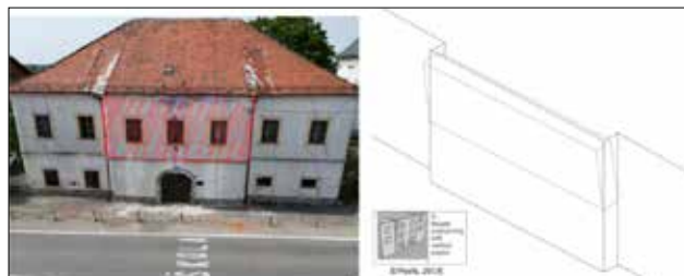
20 Out-of-plane mechanism in the north façade (photo and drawing: Thibaud Maillard, 2023)
