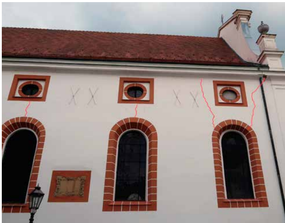
6 General view of the external damage of the church, where there is no evidence of masonry crushing at the anchorage zones of the tie rods (photo: X. Romão, July 2021)
