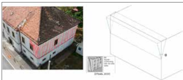
21 Out-of-plane mechanism in the west façade (photo and drawing: Thibaud Maillard, 2023)
