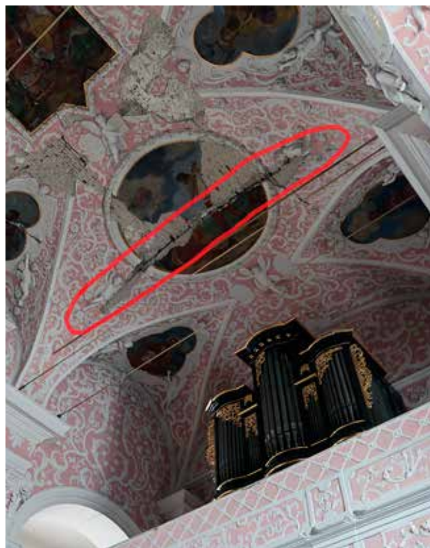
12 Possible constructive joint running along the upper choir arch (photo: X. Romão, July 2021)
