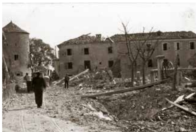
13 Javna cisterna i blok zgrada jugoistočno od župne crkve nakon bombardiranja (izvor: Povijesni i pomorski muzej Istre, PPMI-F-50_IV) Public cistern and block of buildings southeast of parish church after the bombing (source: Historical and Maritime Museum of Istria, PPMI-F-50_IV)
