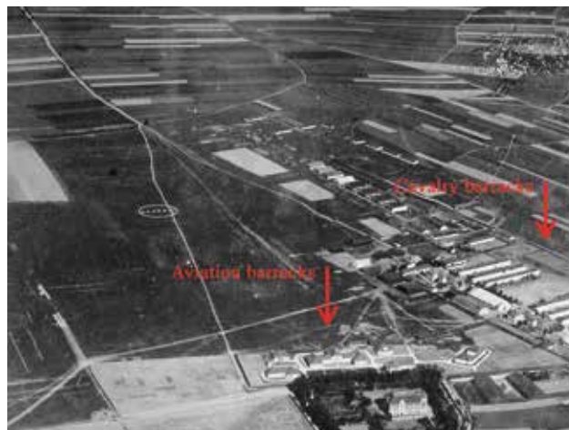
13 Aerial photograph of the Rakowice-Czyżyny airport and aviation and cavalry barracks (MLP, early 1920s).
