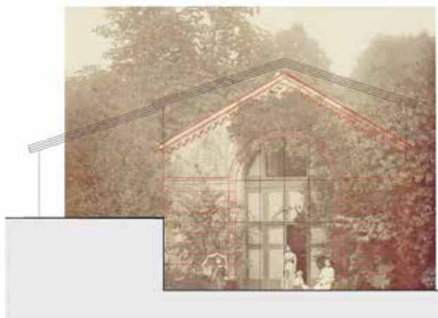
21 Rekonstrukcija spremišta za kočije Reconstruction of the storage facility for carriages
