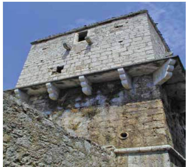
20 Armiranobetonski balkon na Čorićevom tornju (foto: I. Glavaš) Reinforced concrete balcony on Čorić Tower (photo: I. Glavaš)
