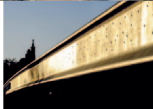
Detail of the J4 footbridge © Lisa Ricciotti
