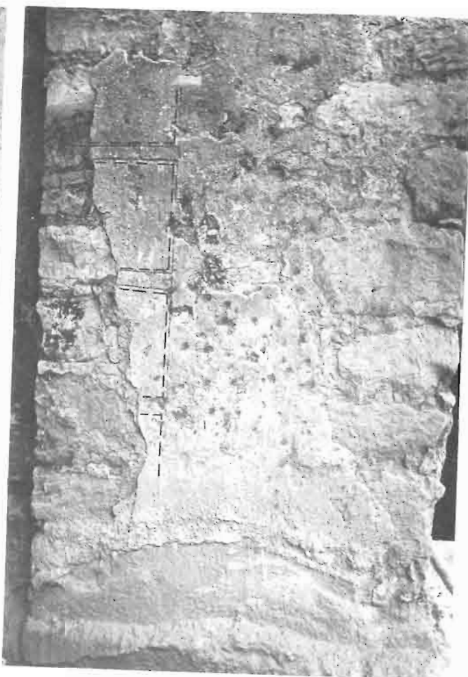
25 Zvonik, naslikani kvadri na pilastru 25 Belfry, painted squares on the pilaster
