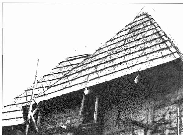
41 Kapela sv. Trojstva, gromobranska instalacija i pokrov kapele, stanje 1982. Chapel of the Holy Trinity, lightning conductor and roof, situation in 1982
