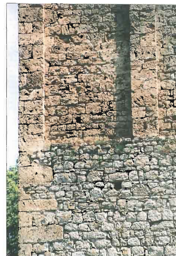
81 Frankopanska kula, struktura lica pročelja Frankopan Tower, structure of the face of the façade
