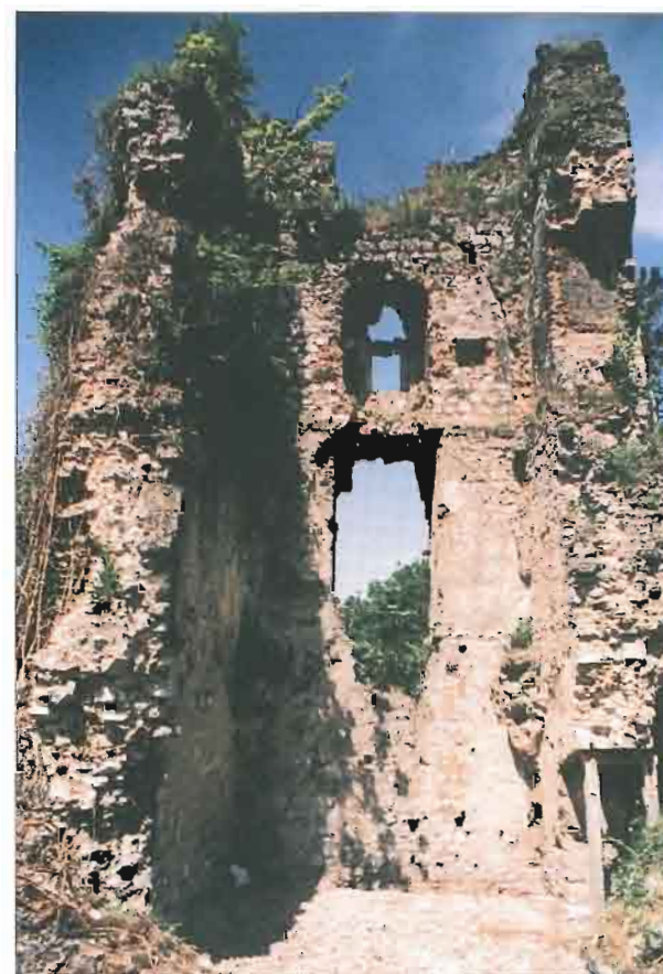
80 Frankopanska kula, pogled s istoka na unutrašnjost kule (1999.) Frankopan Tower, view from the east into the interior (1999)
