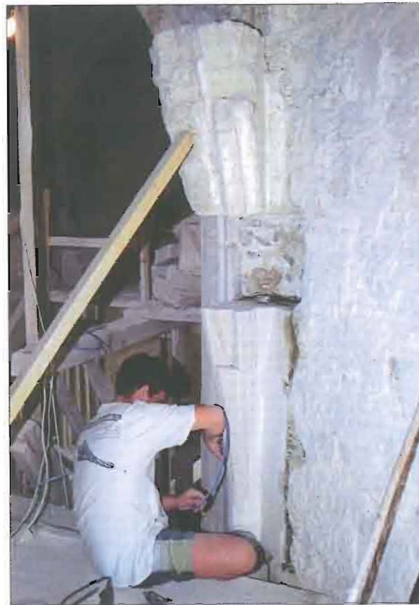
60 Kapela sv. Trojstva, klesanje južne račve svoda Chapel of the Holy Trinity, cutting southern bifurcation of the vault
