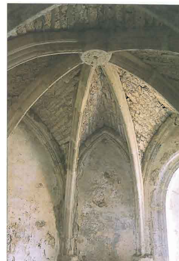
58 Kapela sv. Trojstva, pogled na rekonstruirani svod svetišta Chapel of the Holy Trinity, view of reconstructed vault of the sanctuary
