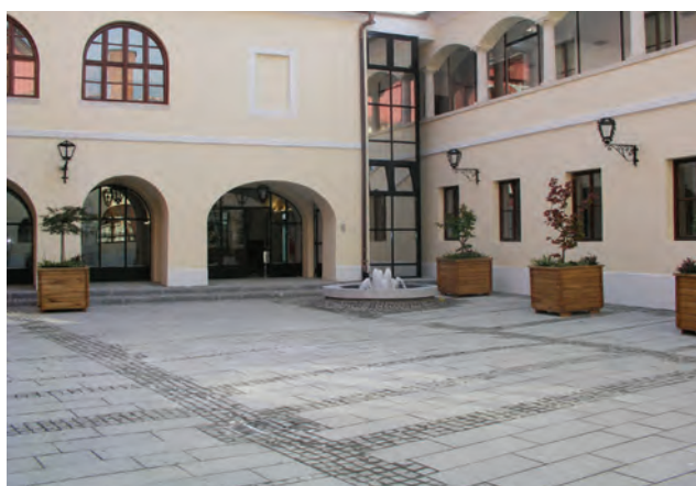
28 Pogled na JE ugao dvorišta (stanje nakon obnove, foto: Željko Trstenjak) View of the SE corner of the courtyard (after renovation, photo by Željko Trstenjak)
