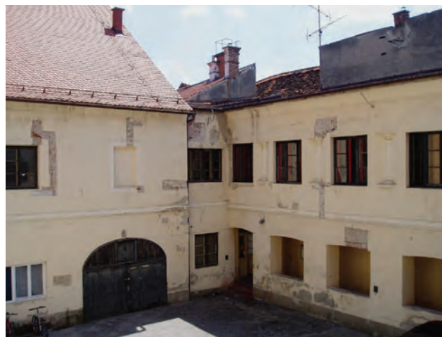
27 Pogled na JE ugao dvorišta (stanje prije obnove, foto: Željko Trstenjak) View of the SE corner of the courtyard (before renovation, photo by Željko Trstenjak)
