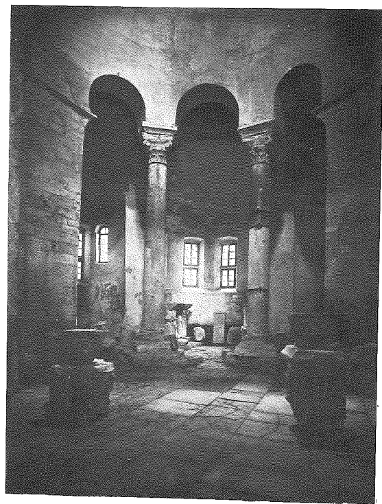
20 Unutrašnjost, pogled prema svetištu, stanje oko 1910. god. Interior, a view of the sanctuary, 1910
