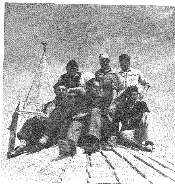
28 Grupa suradnika pri rekonstrukciji krovne građe na tamburu crkve sv. Donata 1958. god. (B. Petravić, Zadar) A group of technicians reconstructing the tambour roofing, St. Donat Church, 1958 (B. Petravić, Zadar)
