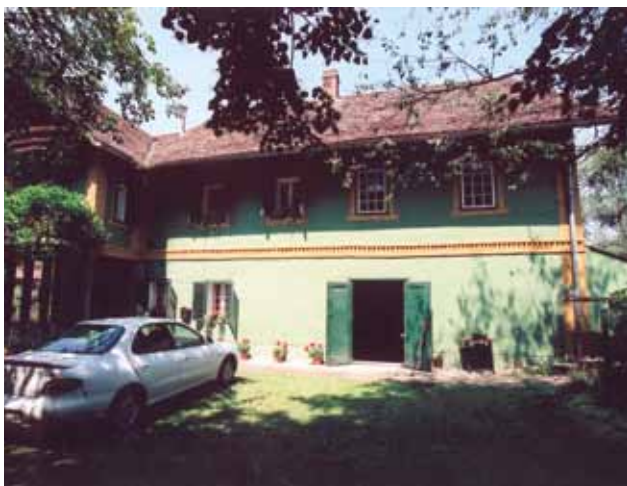
7 Zgrada mlina prije obnove - duže glavno pročelje, stanje 2005. (foto: A. Mlinar) Mill building before restoration – longer main facade, condition in 2005 (photo: A. Mlinar)
