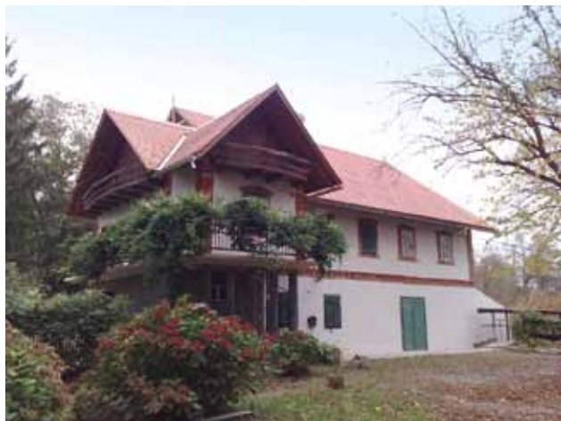
19 Pogled na stražnje pročelje nakon obnove (fototeka Muzeja Moslavine) View of the rear facade after restoration (Photographic Collection of the Museum of Moslavina)
